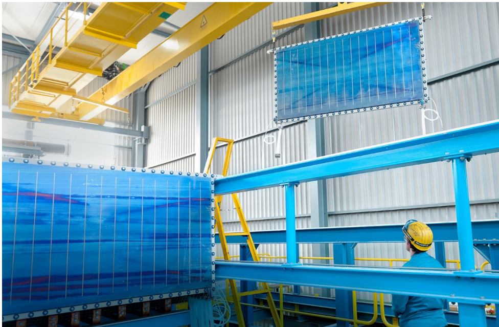
Assembling electrolysis cells
